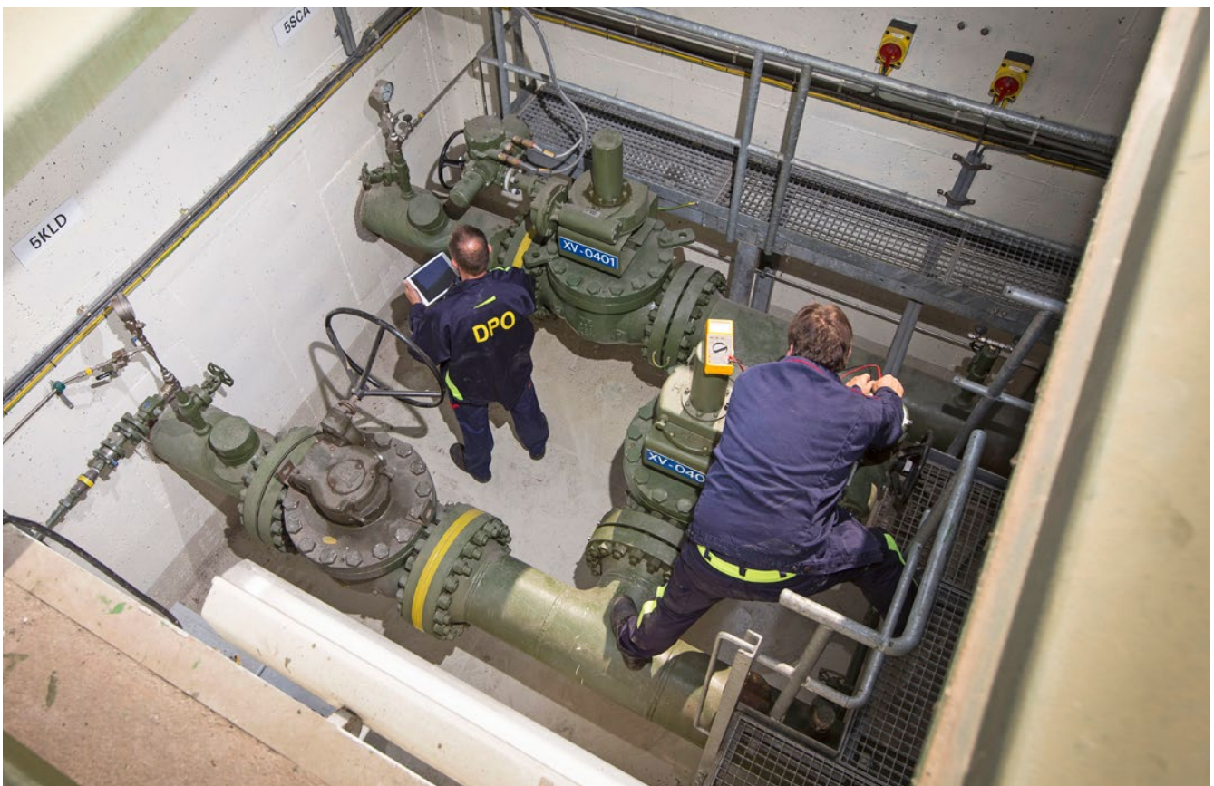
Inspection of one of the valve pits.
